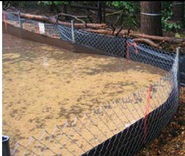
Figure 5.3: Example of Reinforced Silt Fence
