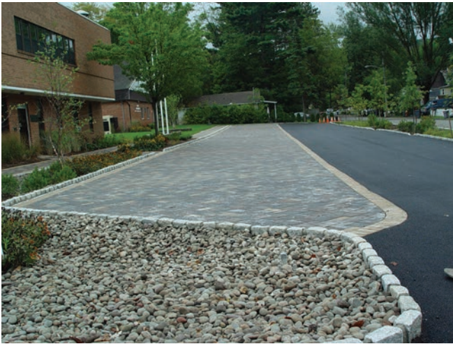
Porous pavers and bioswales adjacent to the municipal building in the Village of Greenwood Lake provide a visible demonstration project. Project funded by the Green Innovation Grant Program. Photo credits: NYS EFC.
