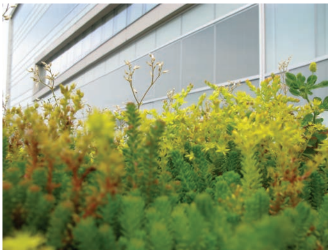
This green roof on the Syracuse Center of Excellence retains stormwater, effectively increasing system capacity.
