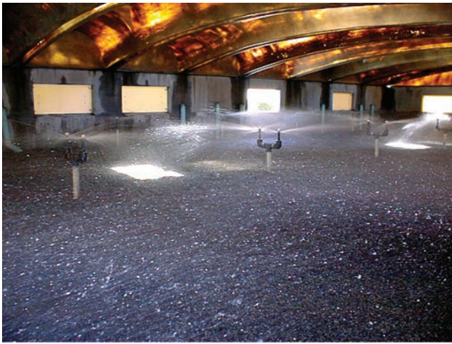
Intermittent sand filter (Secondary Treatment).
