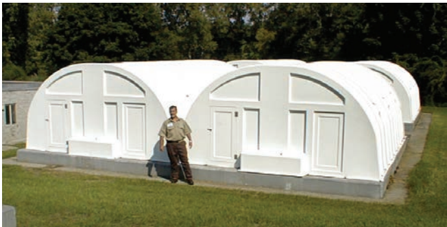
Rotating biological contactors (Secondary Treatment).
