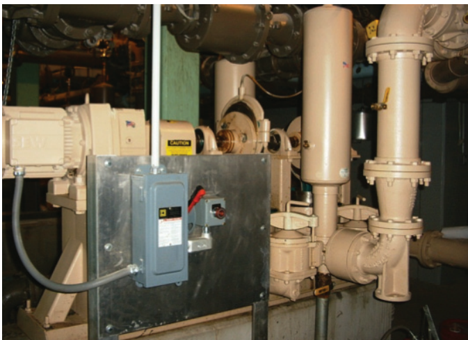
Plunger pump at Lake Placid WWTTP.
