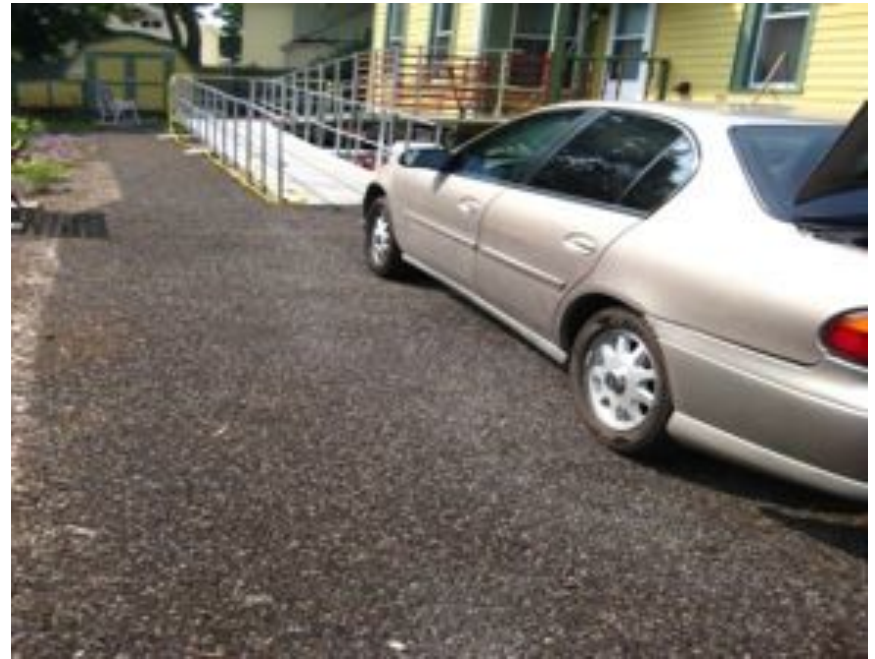
Flexi-pave™ sidewalk and driveway at 515 Tully Street
