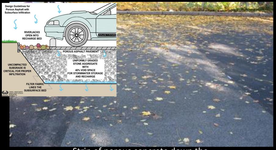
Strip of porous concrete down the middle of an asphalt lot in Syracuse
