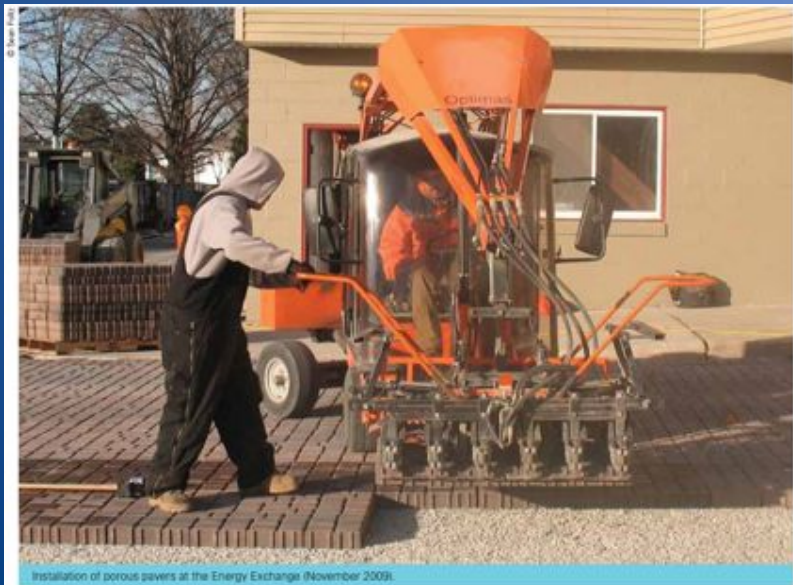
Installation of porous pavers at the Energy Exchange (November 2009).
