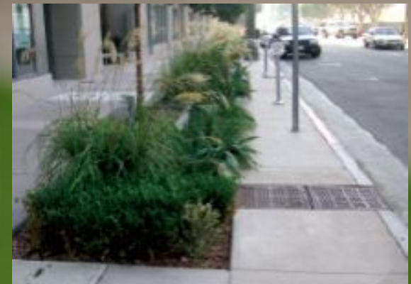
Parkway Infiltration Swale 11 th St & Hope St - Los Angeles
