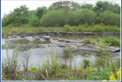
Stream restoration included a series of rock structures for grade control, bank stabilization, enhancements to fisheries and plantings of native species.
