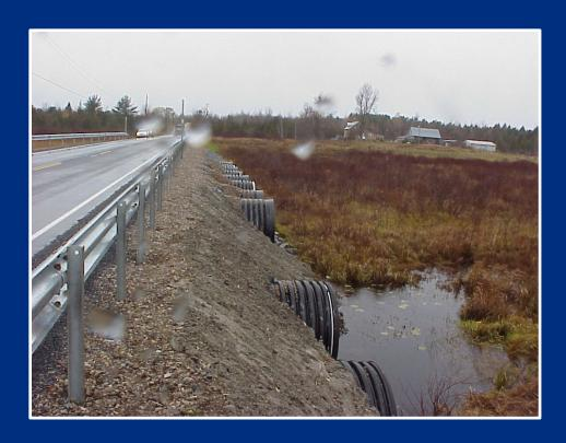
Road was elevated 4.5 feet and increased culvert size.
