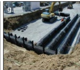
Figure 2: Examples of retrofits employed at small parking lots: permeable pavers (a); dry swale (b); perimeter sand filter (c); grass filter/infiltration trench (d); filter strip (e); internal bioretention (f); underground infiltration (g) and island bioretention (h).
