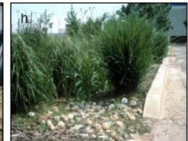
Figure 2: Examples of retrofits employed at small parking lots: permeable pavers (a); dry swale (b); perimeter sand filter (c); grass filter/infiltration trench (d); filter strip (e); internal bioretention (f); underground infiltration (g) and island bioretention (h).
