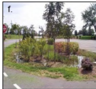
Figure 2: Examples of retrofits employed at small parking lots: permeable pavers (a); dry swale (b); perimeter sand filter (c); grass filter/infiltration trench (d); filter strip (e); internal bioretention (f); underground infiltration (g) and island bioretention (h).
