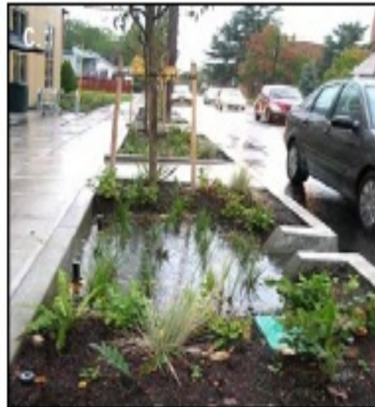
Figure 2: Landscape architects can creatively use stormwater as a resource in foundation planters (a); permeable pavers (b); bioretention (c); and stormwater tree pits (d).
