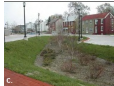
Figure 3: Innovative street retrofits include: curb cuts to rain gardens (a), surface bioretention in traffic calming measures (b), larger bioretention pocket in multi-family residential (c), and curb cuts to cascading bioretention cells (d).
