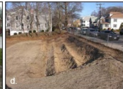
Figure 3: Innovative street retrofits include: curb cuts to rain gardens (a), surface bioretention in traffic calming measures (b), larger bioretention pocket in multi-family residential (c), and curb cuts to cascading bioretention cells (d).
