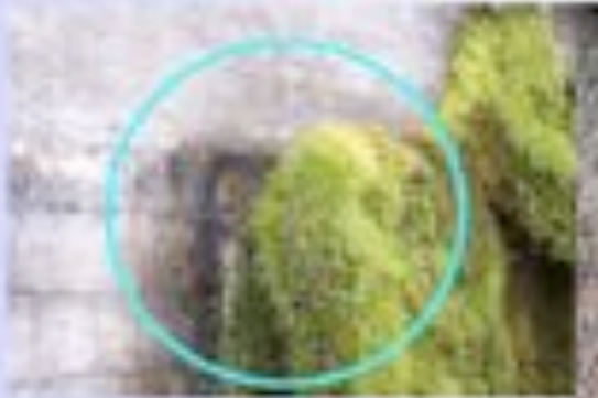
Leaking reservoir wall
