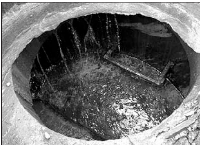
Groundwater infiltration makes efficient treatment difficult.
