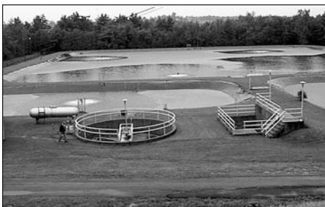
Aerated lagoons are secondary treatment processes.
