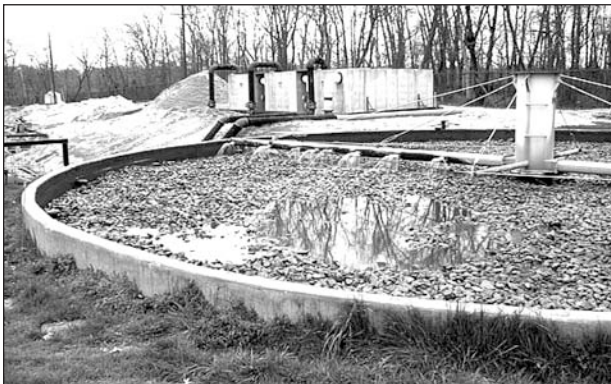
Fixed film and old trickling filter stone, above, are sometimes replaced with more efficient plastic media, right.
