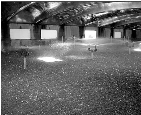
Intermittent sand filter (Secondary Treatment)
