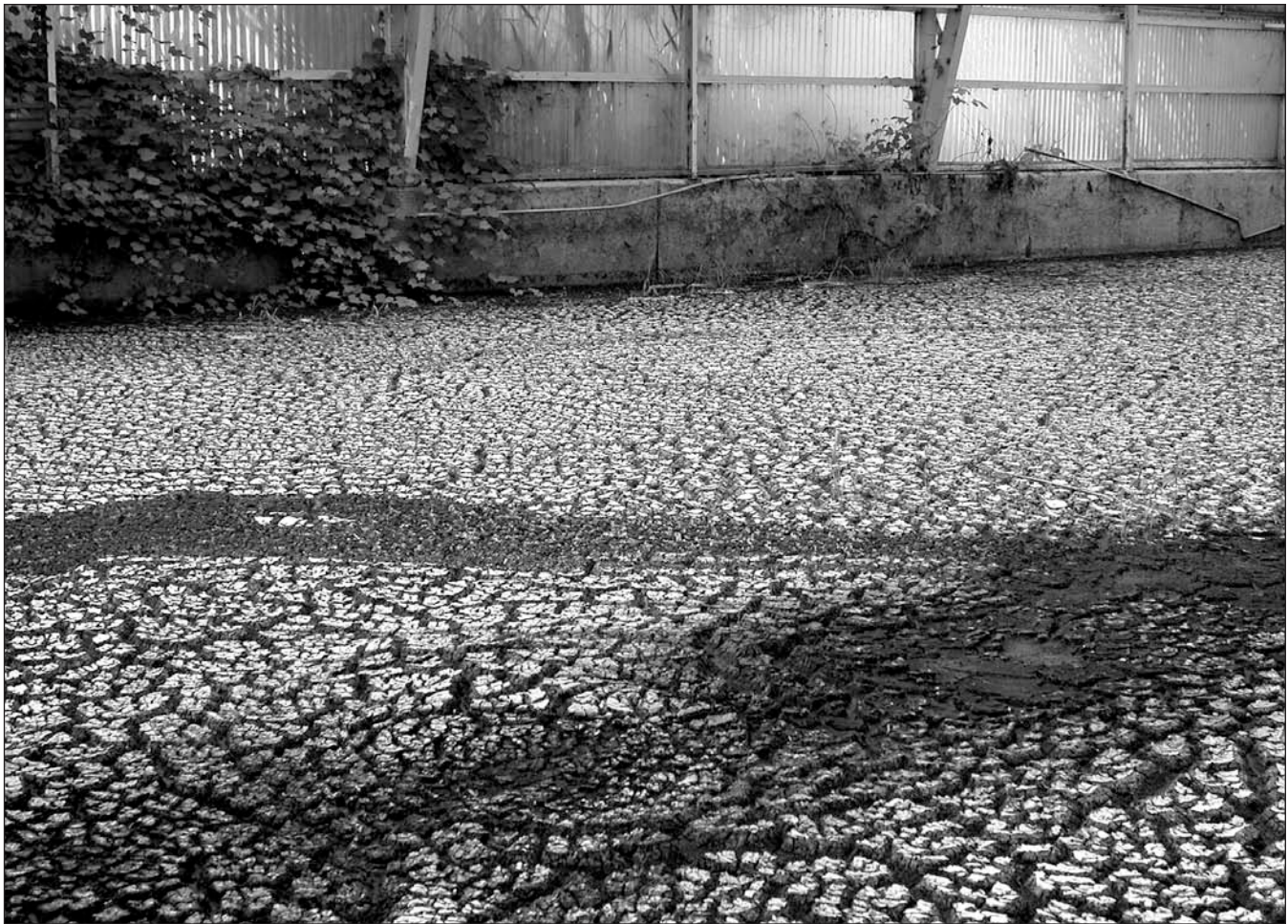
Sand drying beds can be problematic, particularly with rainy conditions.
