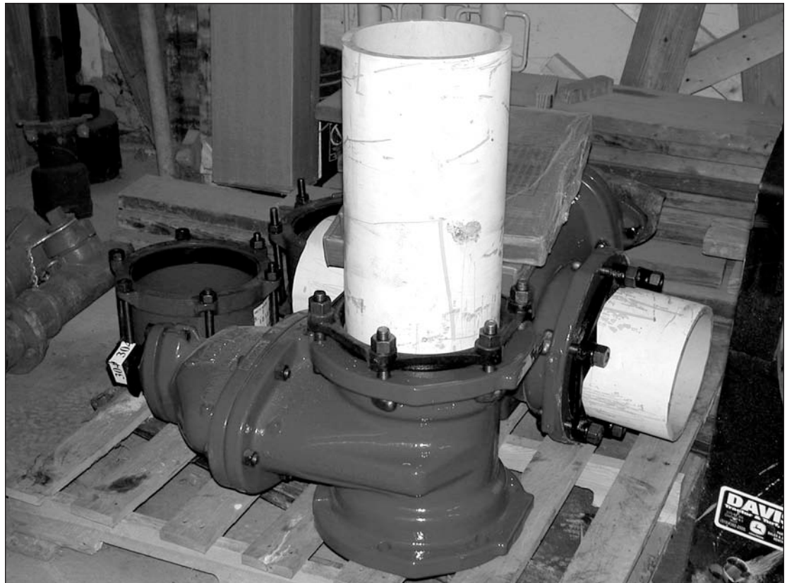
Replacement valve with preassembly awaiting installation
