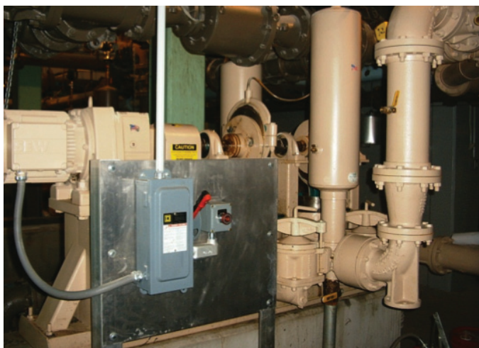
Plunger pump at Lake Placid WWTTP.
