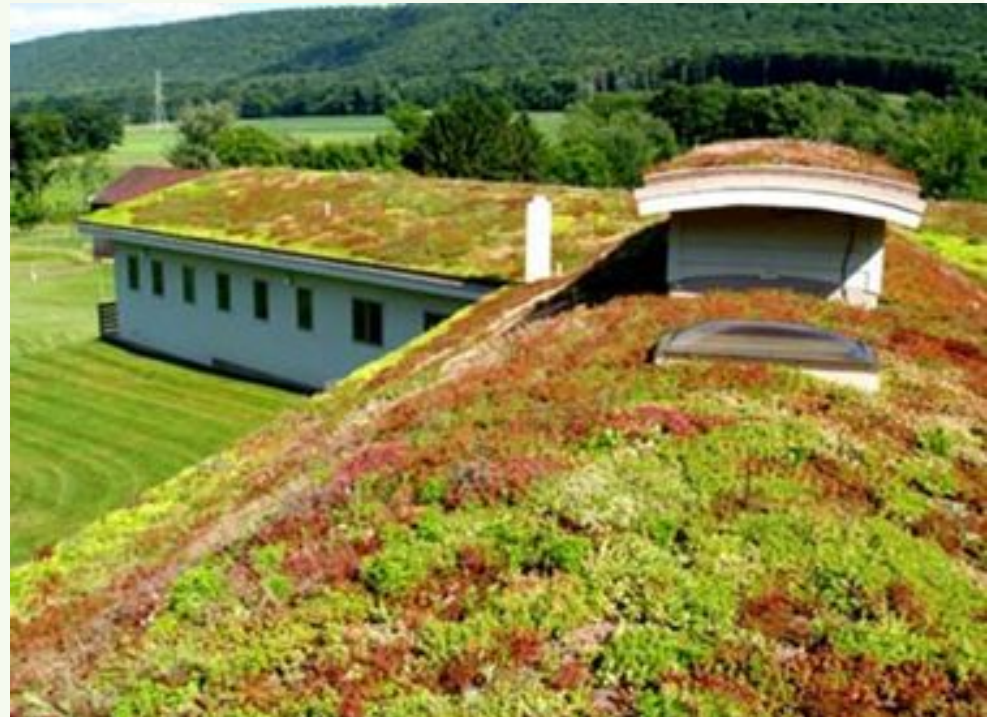
Extensive green roof. City of Windsor, 2009.
