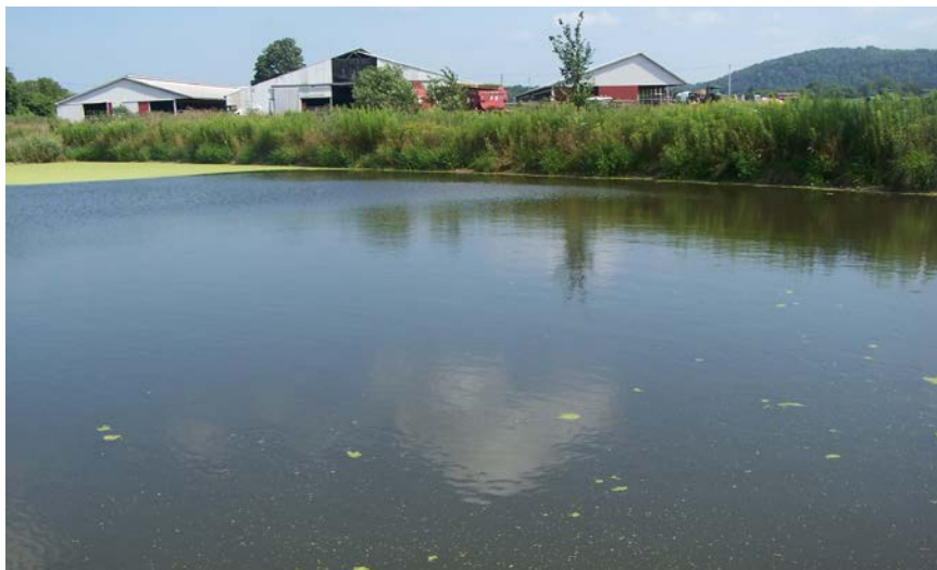
A single filter cell shows the detention capacity of the wetland.
