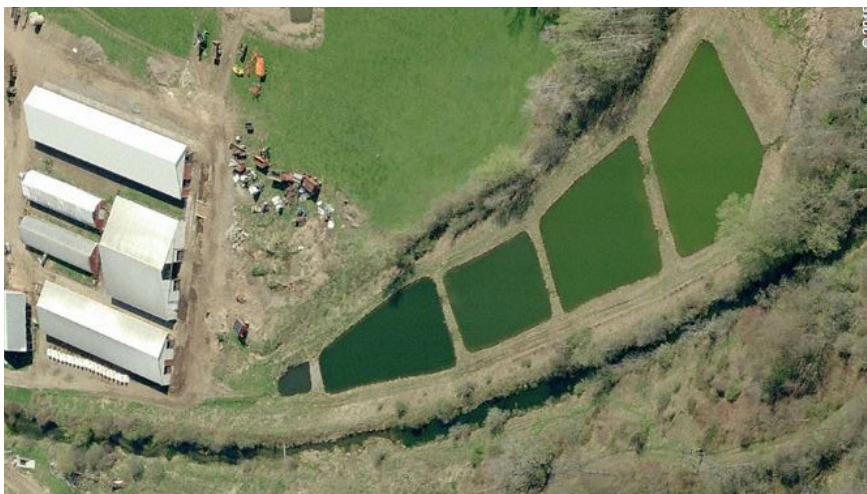
The wetland was separated into five segments to allow retardation of water flow, which prolongs biological activity and enables sedimentation to improve water quality.
